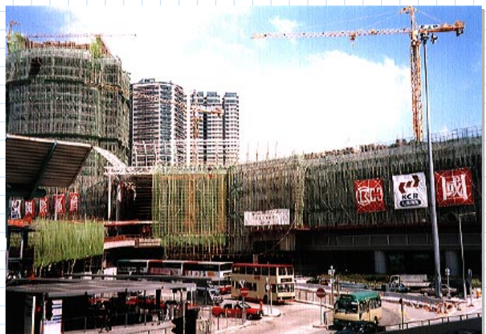
Hung Hom Station under Reconstruction
